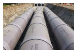
Reinforced plastic composite pipes are also used as rainwater storage pipes
